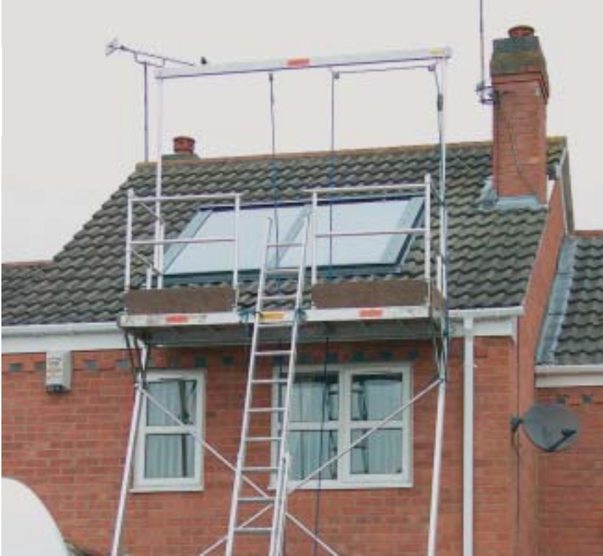
Attaching the solar panel
