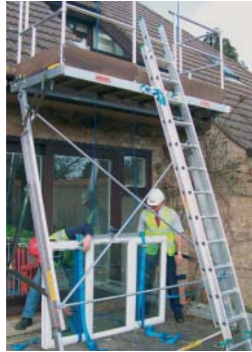
Attaching the new window
