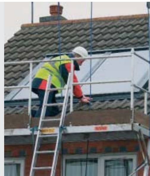
Solar panel in position
