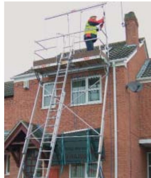
Hoisting the solar panel
