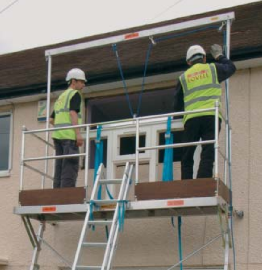
Attaching the new window
