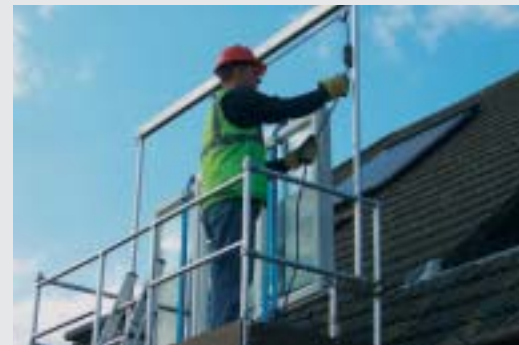
Hoisting to final position
